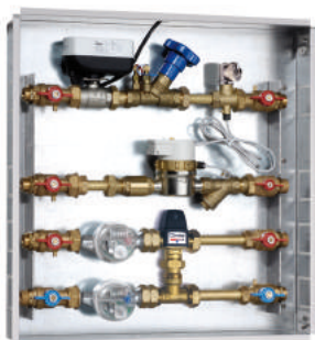
482 - 1 DHW/DCW mixing valve
