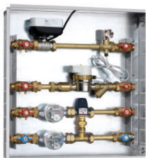
472 - 1 DHW/DCW mixing valve
