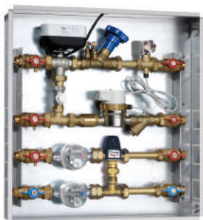
483 - 1 DHW/DCW mixing valve
